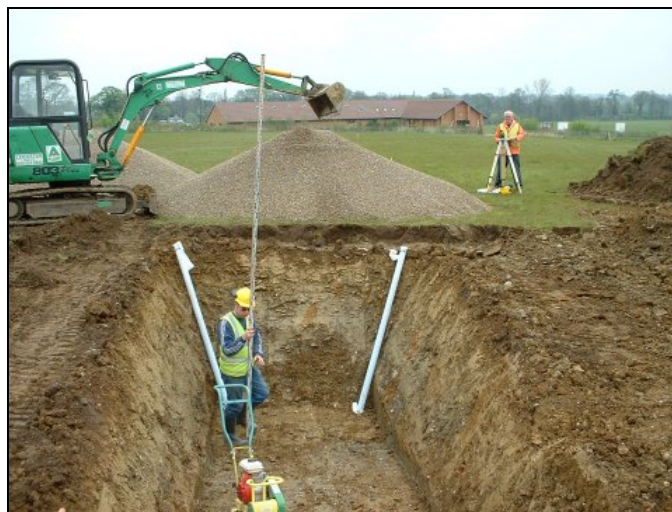
Construction of the Radar test pit, April 2002
